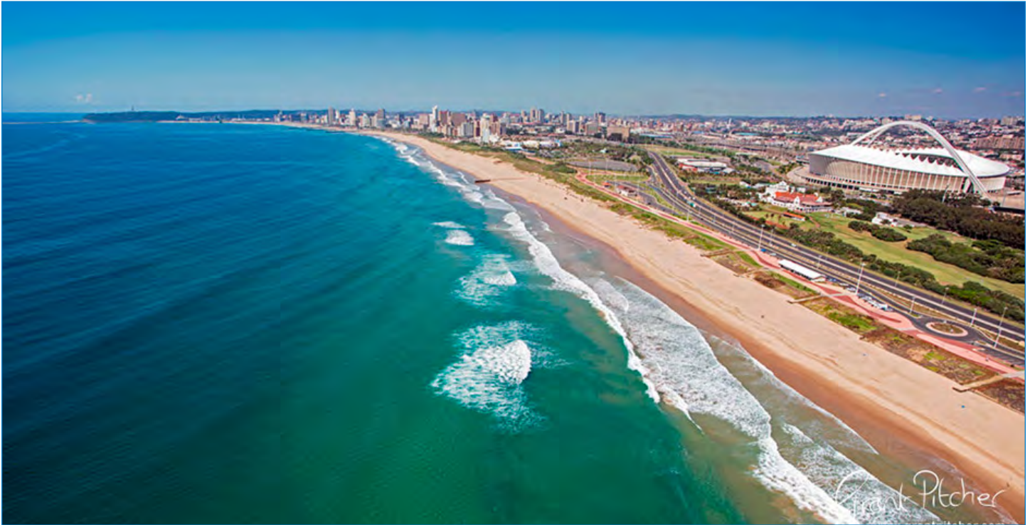
Aerial view of the Durban, South Africa coastline (courtesy of Grant Pitcher)
